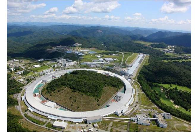
SPRING8, 1999, Japan: 8 GeV, 1436 m ring, 48 beamlines
