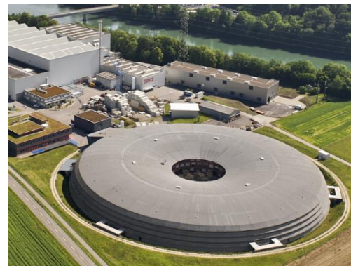
SLS, 2001, Switzerland: 2.4 GeV, 288 m ring, 16 beamlines, to be upgraded to DLSR during 2023-2025
