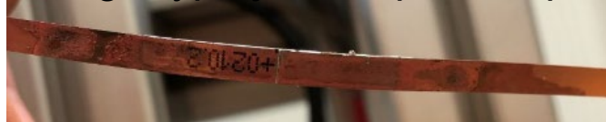
bridge-type joint: tape-to-tape
