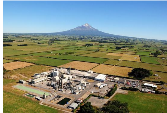
Planned electrolyser plant for green urea production for fertiliser
