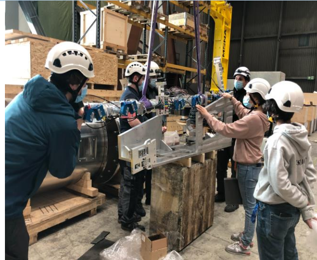
Large bar preparation and installation at b.191
