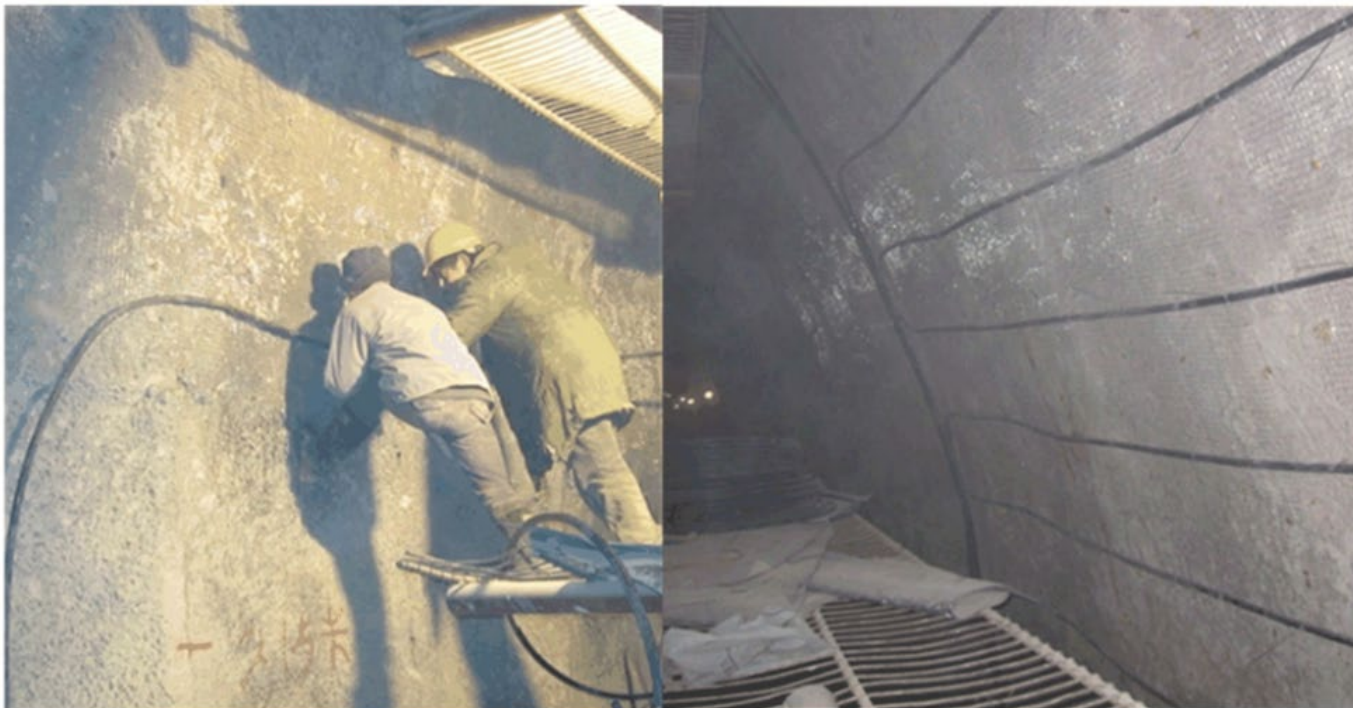
Fig. 2. Installation of tunnel lining GHEs at Linchang tunnel.
