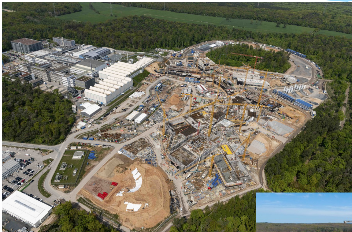
FAIR- Construction Site (May 2022)
