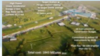
ESS (0.8 GHz) (under construction)
