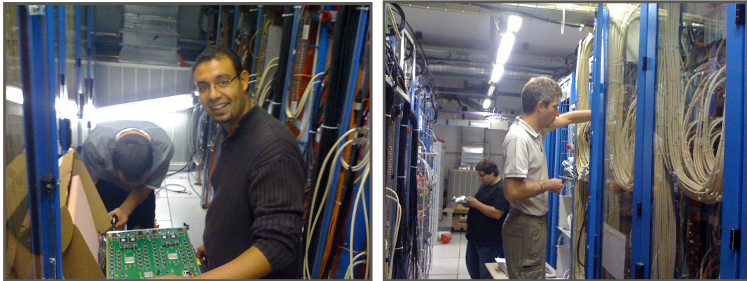
TCC Installation (September 2009)
