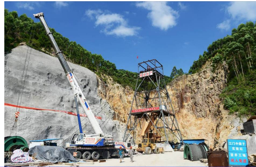
~ 600m vertical shaft, ~1300m sloped tunnel All blasting completed on Dec. 30, 2020, water pool construction on the way
