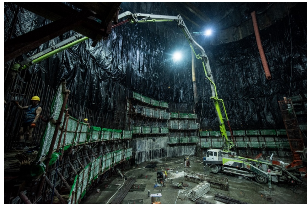
~ 600m vertical shaft, ~1300m sloped tunnel All blasting completed on Dec. 30, 2020, water pool construction on the way
