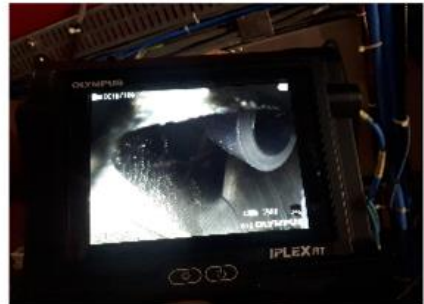
Cut bypass pipe RB3/RB4
