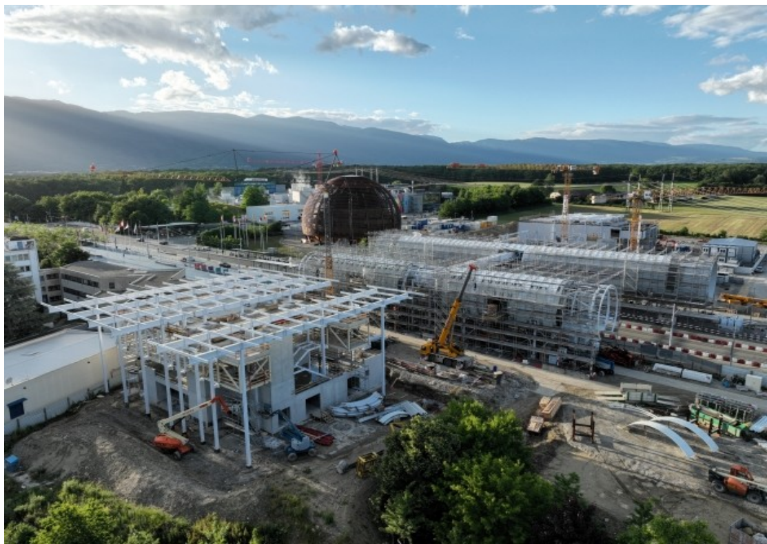
Construction of CERN Science Gateway
