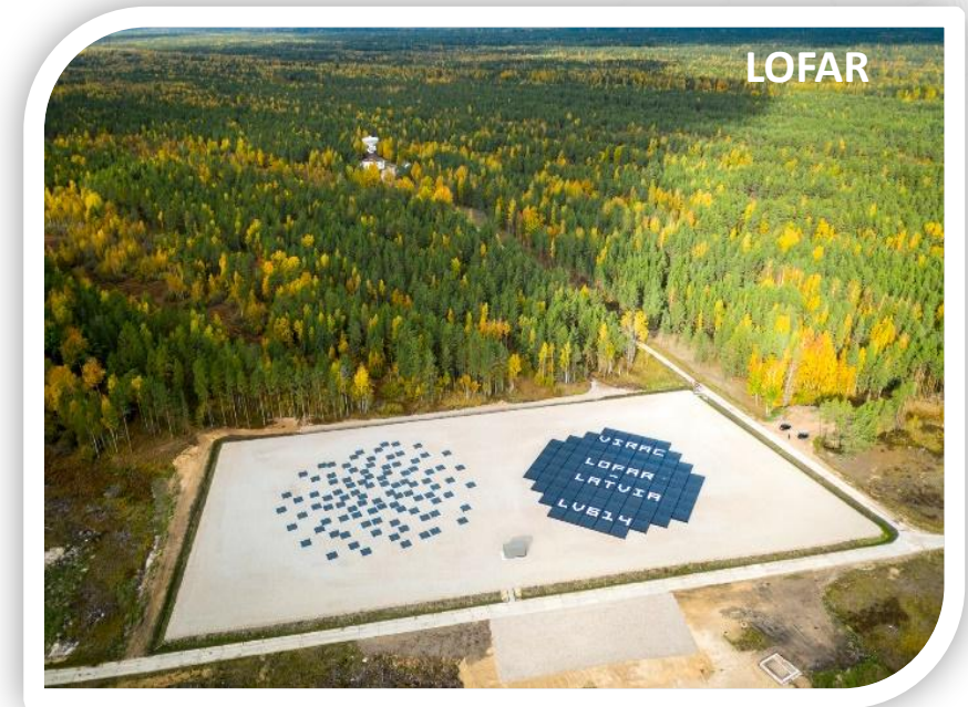
LOFAR station (LV614) 96 antenna array for low freq. obs., 96 antenna array for high freq. obs.
