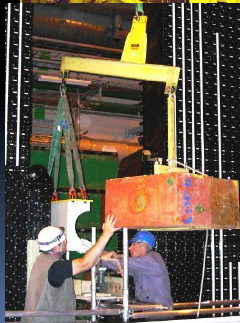
Beam plug installation
