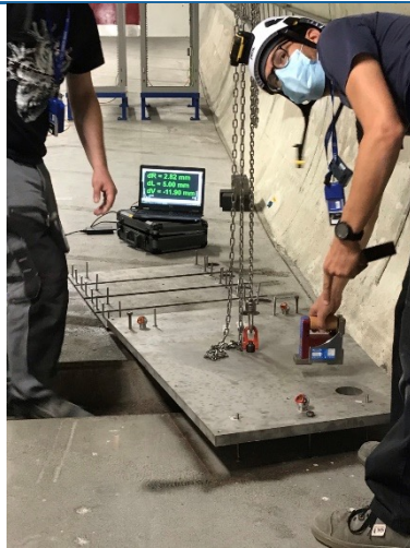
Survey and positioning of baseplates for muon filters
