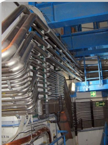
Installation of about 34 Km of austenitic stainless steel for LHC accelerator - CERN
