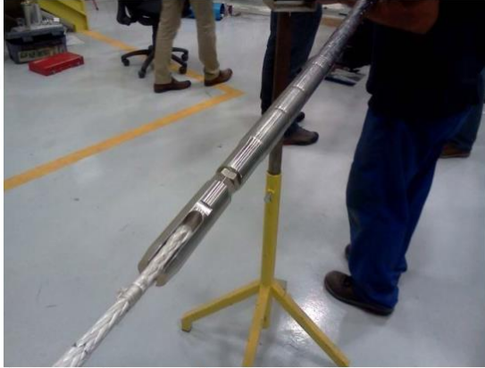
Figure 4.a) The connection between the pulling rope and the cable
