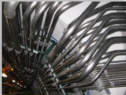
Installation of about 34 Km of austenitic stainless steel for LHC accelerator - CERN
