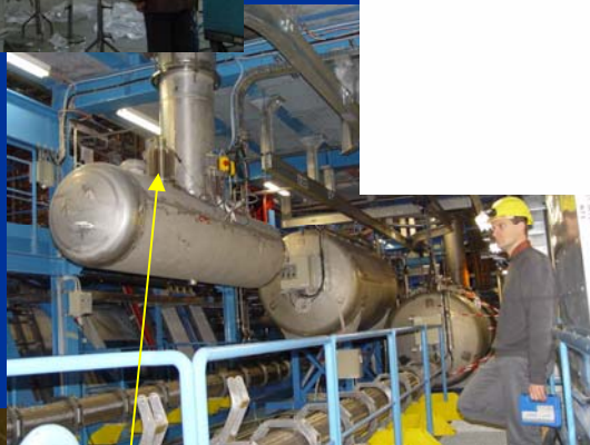
Phase separator cryostat for Toroids
