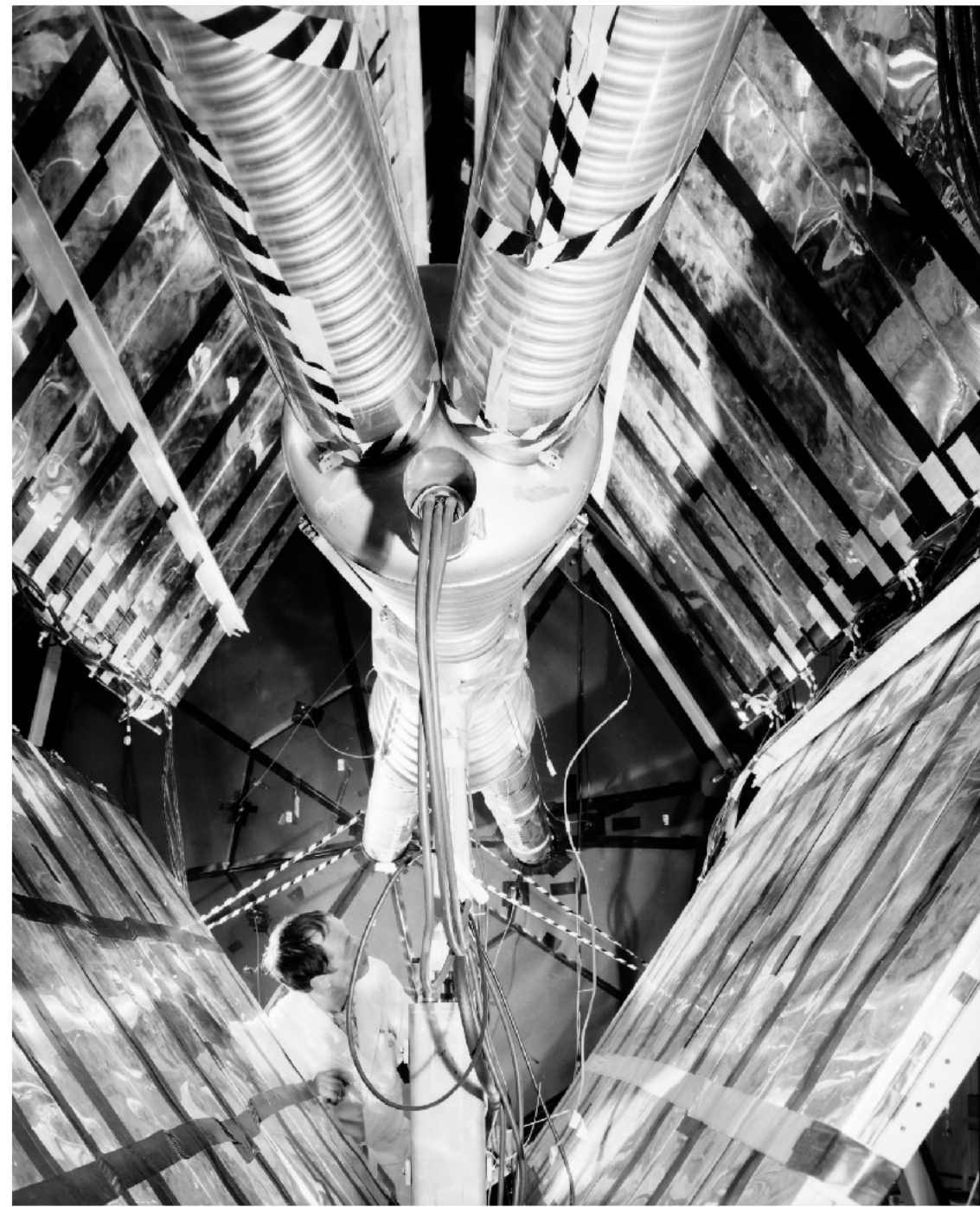
A vacuum chamber where the proton beams collide in the ISR http://cds.cern.ch/record/41966
