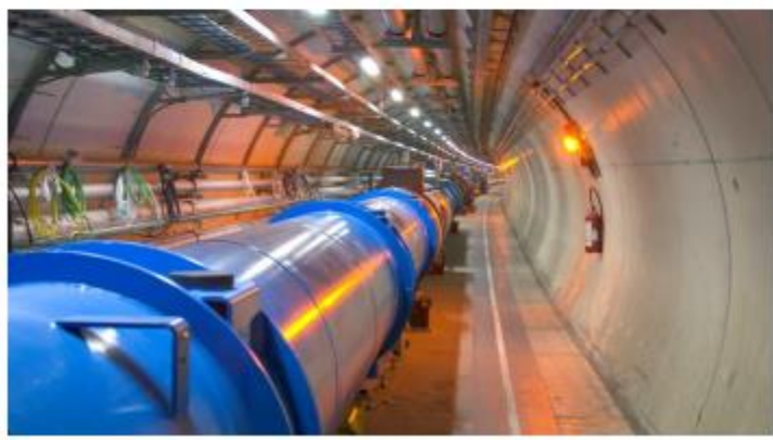
LHC tunnel (27 km)
