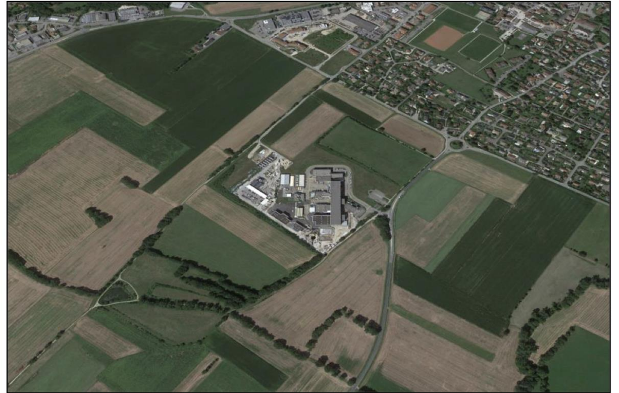
Typical existing semi-rural location – LHC Surface Site
