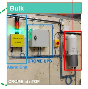
Uninterruptible Power Supply Includes a battery for continuous operation
