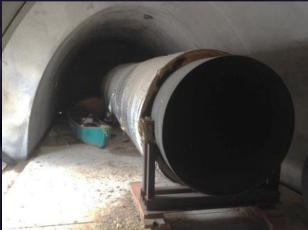
8m section of beamtube in storage at LLO ~ 20 yr
