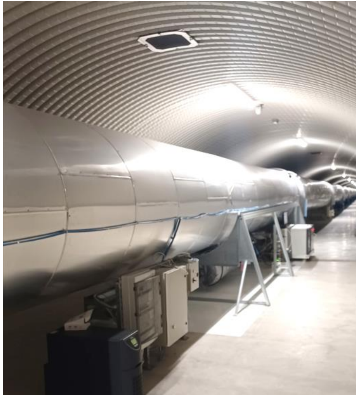
III. Pumping stations @ \approx 0 V
