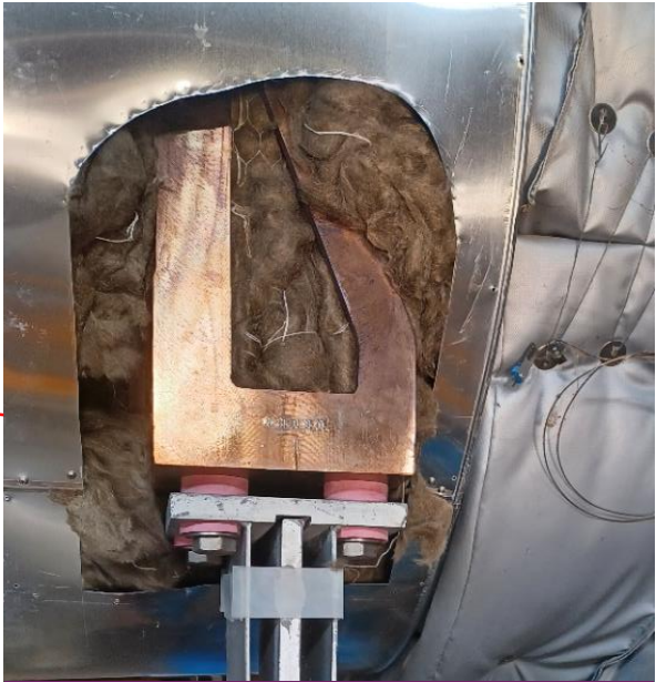
I. Electrical isolation of beampipe stands &
