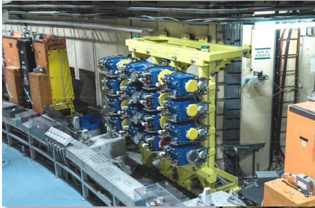
Newly installed H- injection
