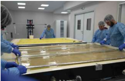
LM2 Drift Panel Construction
