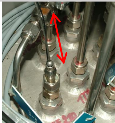
Insertion Thermometer Example: LHC QURC, wire with alignment balls
