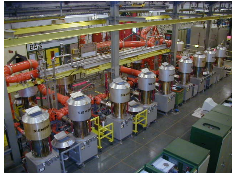
CERN SPS, RS 2004 Tetrode, Trolley (single amplifier), and transmitter (combination of amplifiers) Two transmitters of eight tubes delivering 2 \times 1 \text{ MW} @ 200 MHz, into operation since 1976
