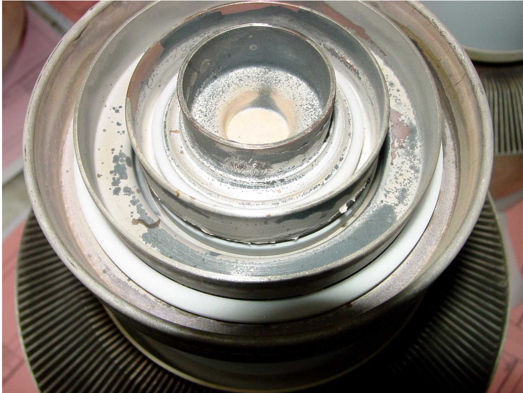
Overheating due to lack of air cooling
