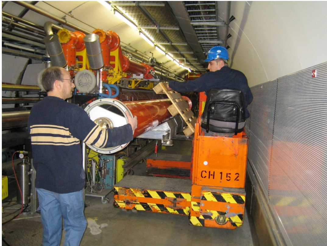
Transporting a piece of 5 meters of a 345 mm Coaxial Line
