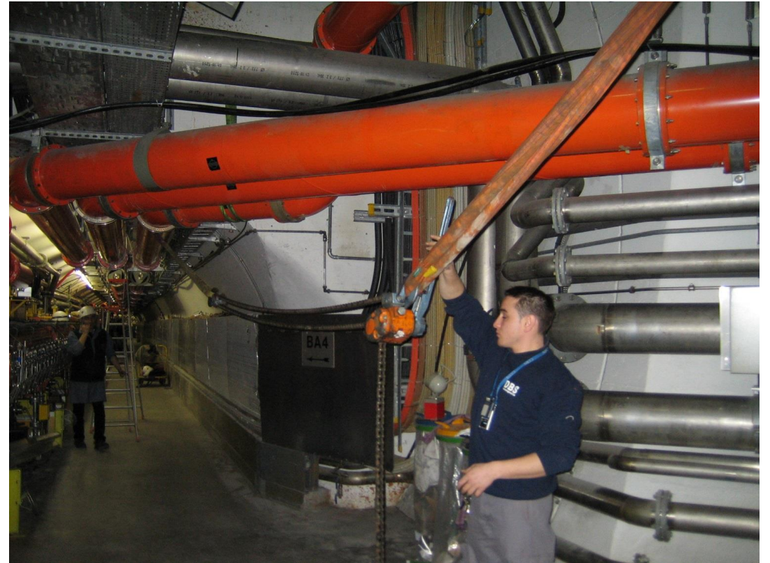
Using a crane to join two 345 mm Coaxial Line
