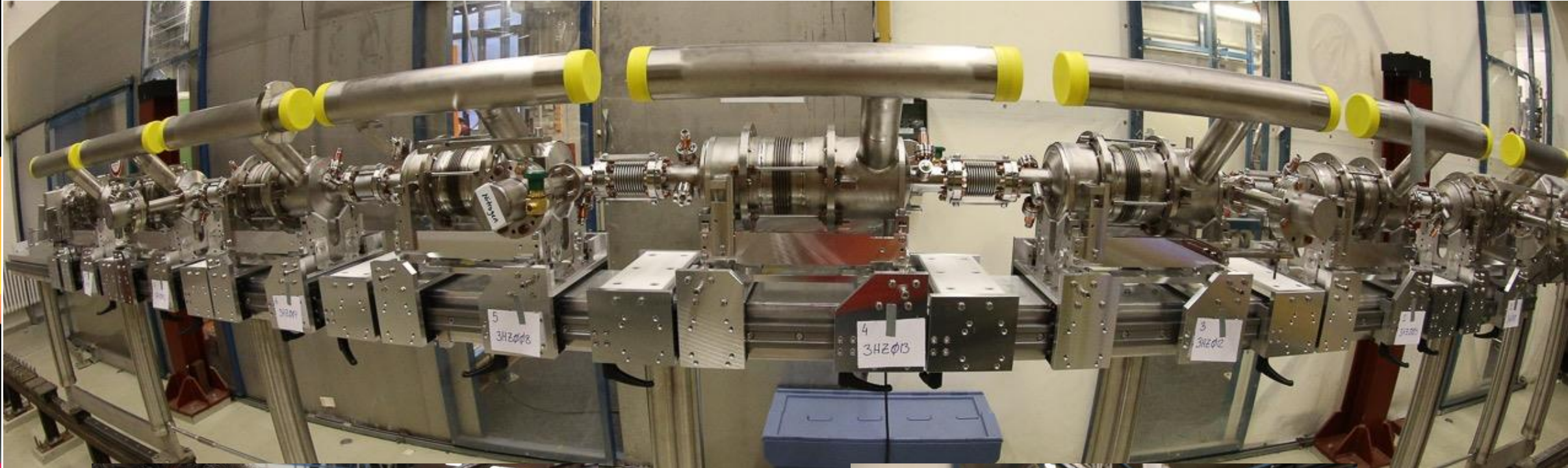
Ti welds to complete cryogenic circuit of cavities
