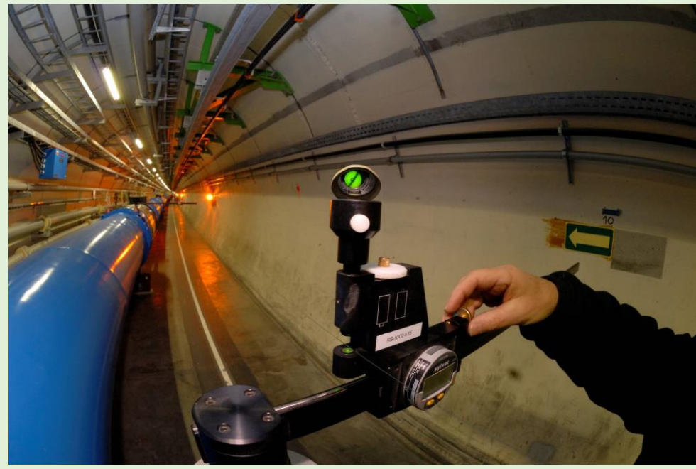
Wire protection pipe
