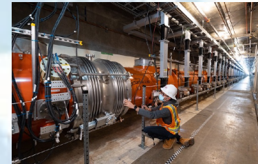
LCLS-II-HE (under construction)
