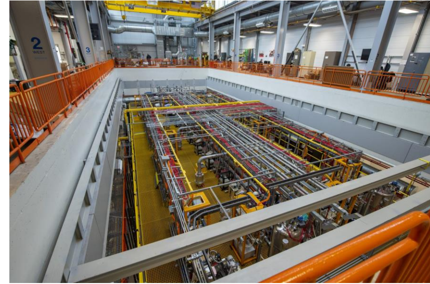
Cryostat before overburden, CRT installation
