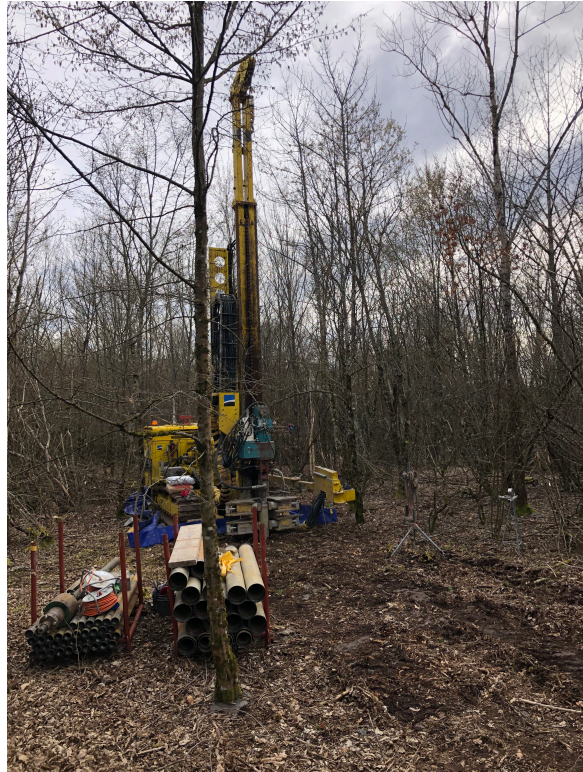
➤ Drilling machine in place
