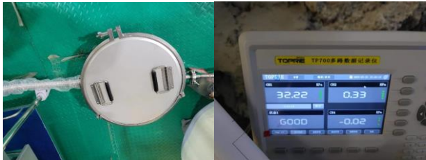
Leakage test after installation
