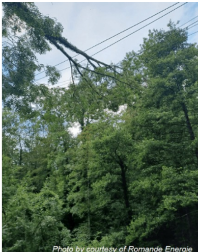
Photo by courtesy of Romande Energie
