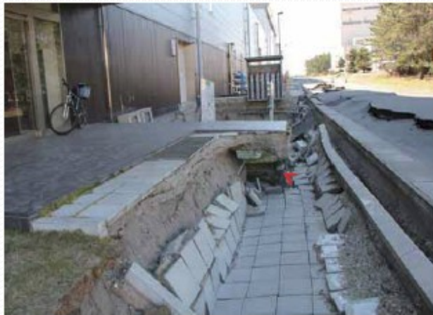
Linac building entrance (J-PARC)
