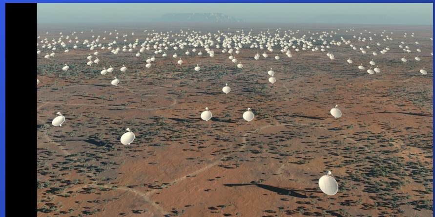
Artist's impression of the 5km diameter central core of Square Kilometre Array (SKA) antennas.
