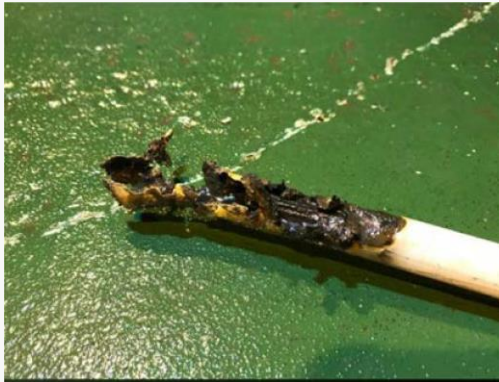
WACS Cable (shunt fault – 2020) in Africa
