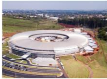
Oct 2018 Building ready
