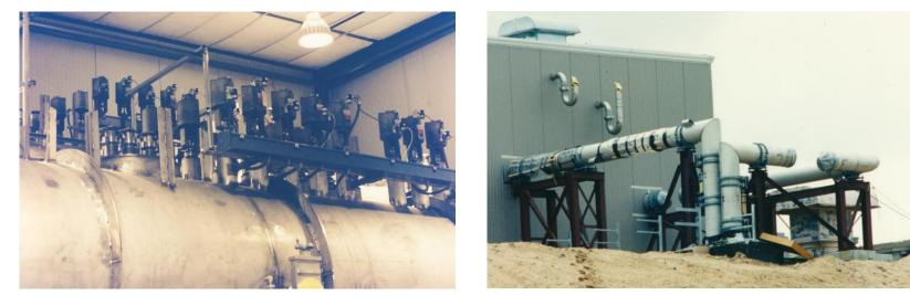
The two CCB cables (one dipole, one quad) start at the valve boxes in the equipment houses outside the ring. They are pulled through the VJ piping, which enters the ring through access openings.
