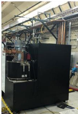
New 50 MW peak power C-band klystron installed in September 2019
