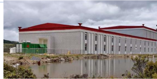
The small on-site Data Center at Daocheng (altitude 4500m).
