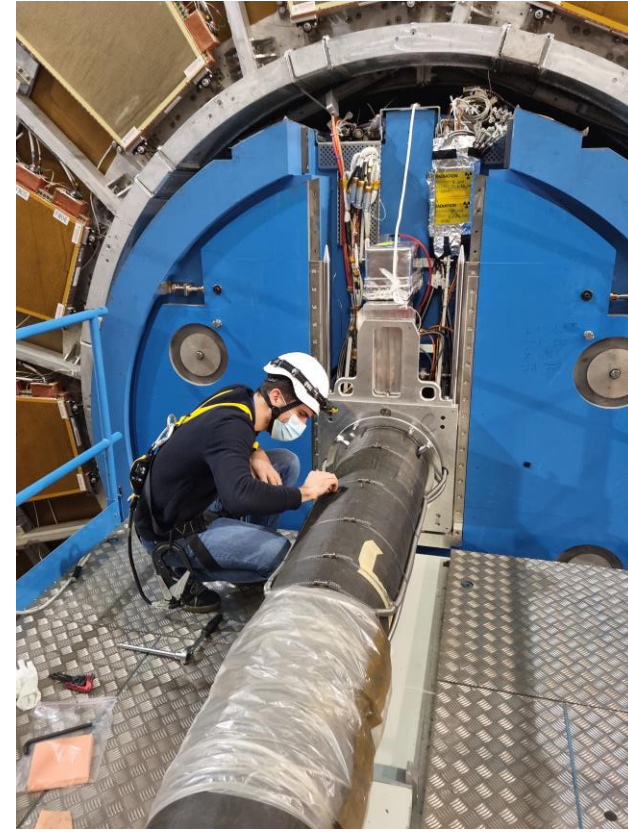
Installation of the VT and VJ aluminum chambers
