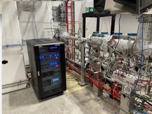
Local vacuum controls rack
