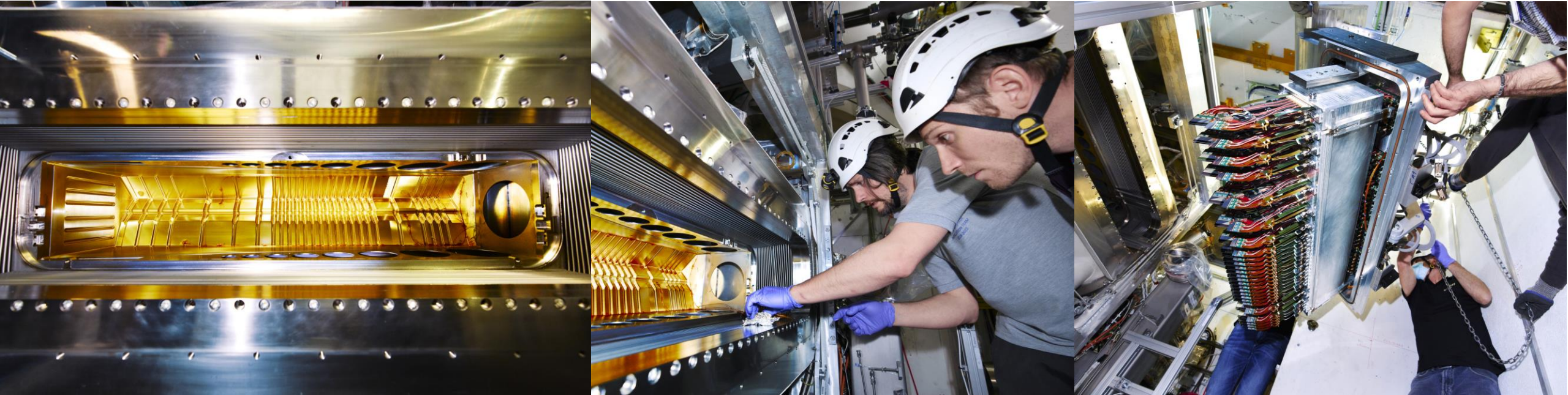
Installation of the VELO A-side
