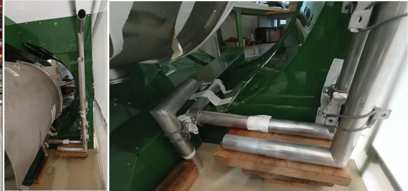
Temporary integration of pumping lines in mock-up. Adjustable system.
