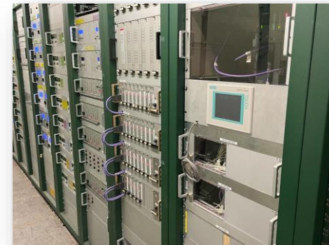
IP2/3 compliant racks – Plexiglass covers to see the PLCs
