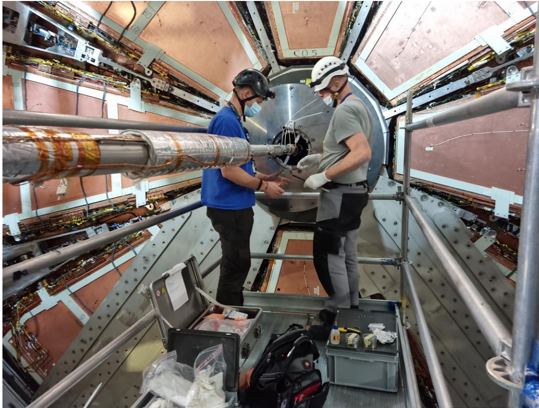
Installation of the VT and VJ aluminum chambers
