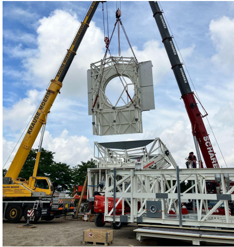
Construction of the LAT at Vertex in Germany
