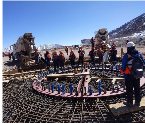
Pouring of the foundation of the LAT platform at the site
