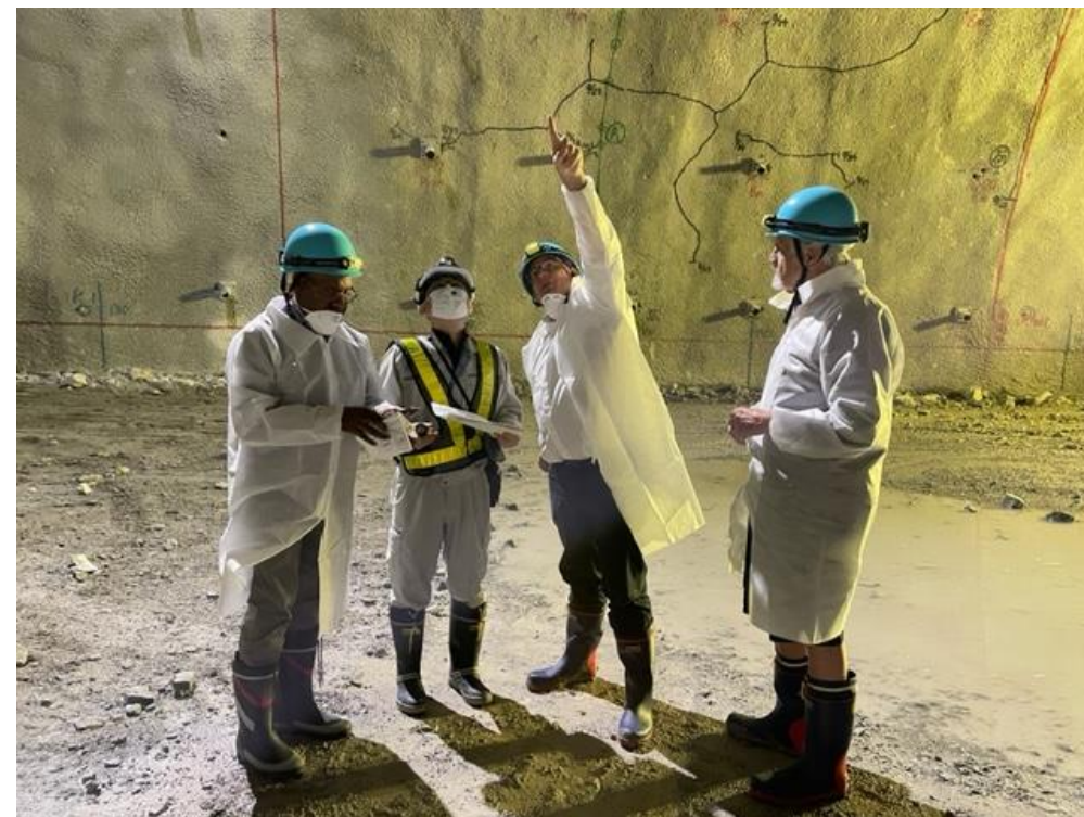
Zinkgruvan Mine Manager Craig Griffiths (pointing upwards) visiting the Hyper-Kamiokande excavation site on 27 Sept 2023
