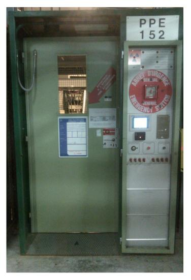
Installation of a new access system as the one installed in the PS experimental areas (i.e. PS AD and East Hall)
