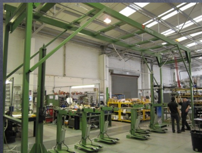
Holding frames for Bus Bar handling during taping
