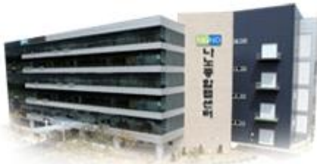
8 inch fabrication line
