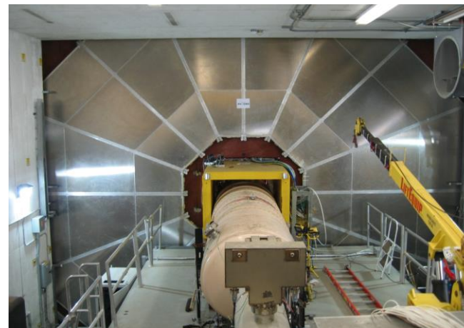
RPC3S - installation (Sep. 22 nd , 2010)
