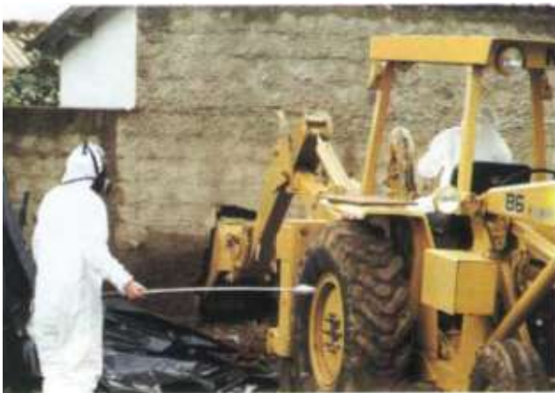
10. A hole is made to remove a radiation hot spot giving a dose rate of 0.5 \text{ Sv}\cdot\text{h}^{-2} .
